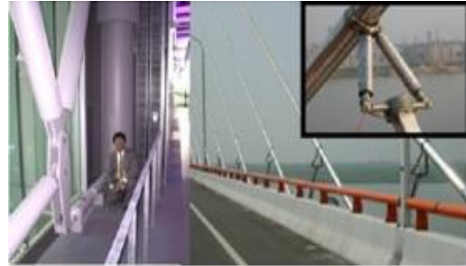
Fig 5. Dongting Lake Bridge, China
