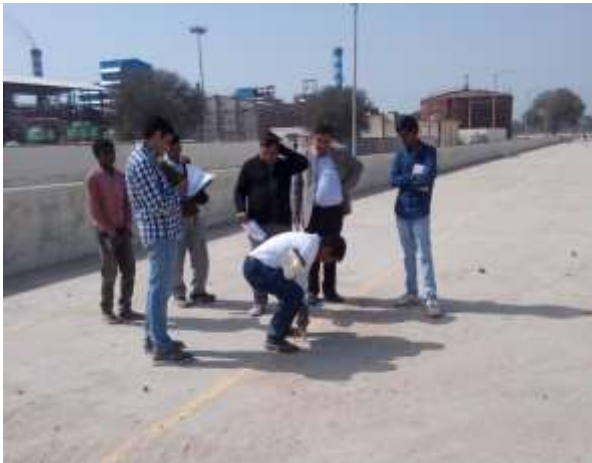
P7 RH Testing of Floor Slab
