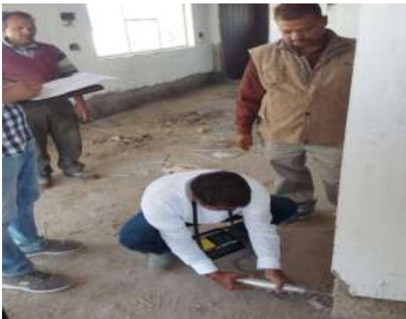
P8 RH Testing of Un-plaster Column Surface
