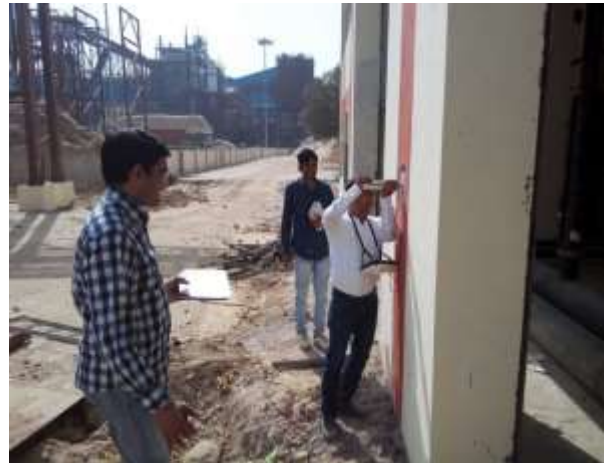
P3 RH Testing of Un plastered Column
