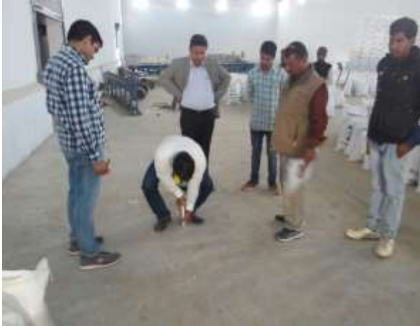
P6 RH Testing of Floor Slab
