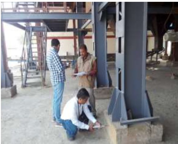
P1 RH Testing of Column Foundation
