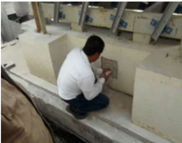
P 2 RH Testing of Foundation Block
