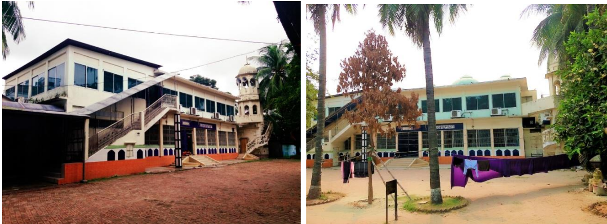
Figure Shows:: Extended new mosque construction adjacent to Bibi Maryam Mosque.
