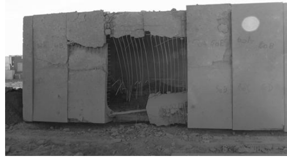
Figure6: Breaching failure due to a close-in explosion of 6000kg TNT equivalent
