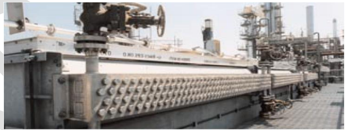
Figure 6. Header-box of an air-cooled heat exchanger
