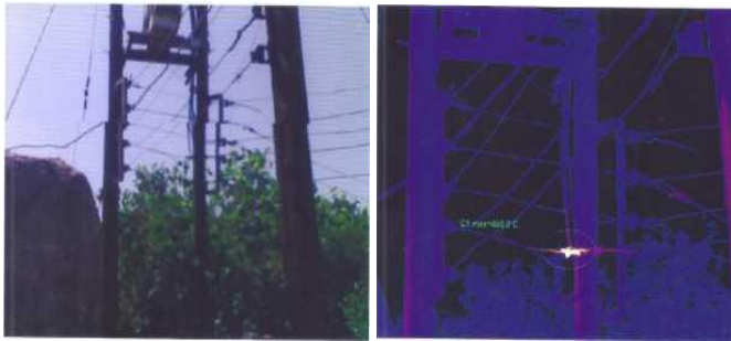
Fig. 3 Normal and thermal picture of weak connection in electricity distribution network
