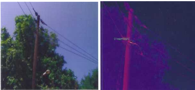
Fig. 4 Normal and thermal picture of molten in parts of the conductor in distribution lines
