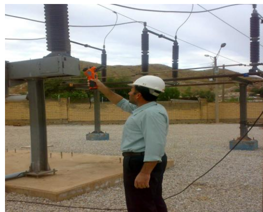
Fig. 10 infrared camerawork using Hot Find LXS camera model
