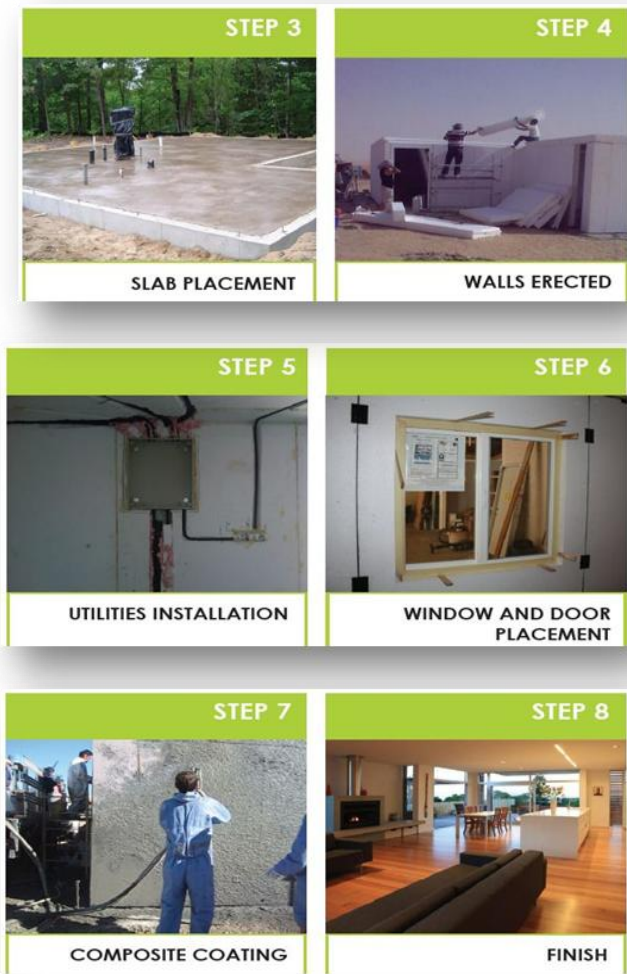
Figure 2: steps of construction of a house using schnell technology
