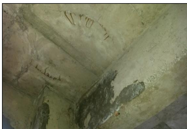
Fig. 3. Honey combing hidden with cement paste, slab leakage, uneven slab surface with rust stains clearly visible
