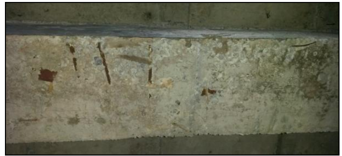
Fig. 8. Beam bottom found with piece of wood and honey combing
