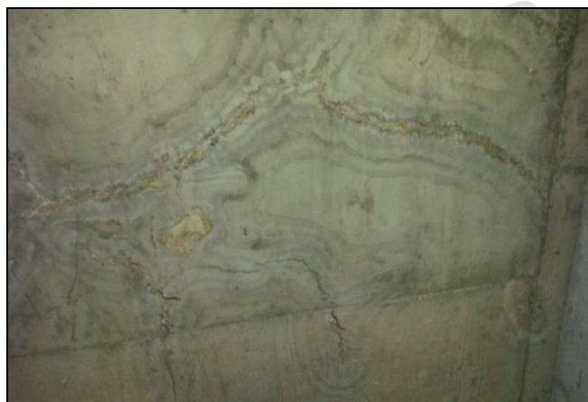
Fig. 2. Excessive leakage with rust stains visible at slab bottom
