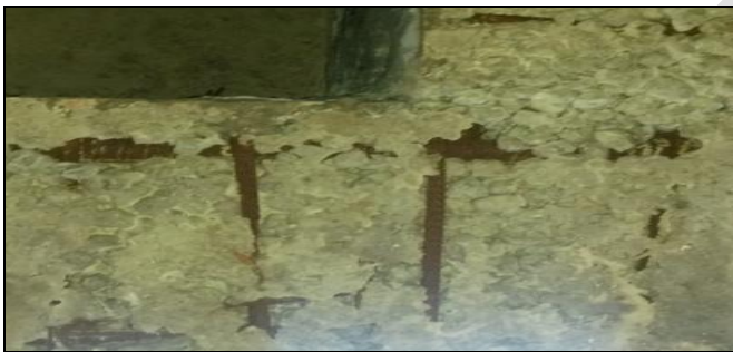
Fig. 5. Beam-beam junction badly affected by loss of cover, honey combing and exposed reinforcement
