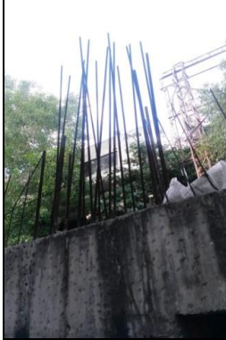
Fig. 9: Column affected by severe honey combing, hidden by cement paste Fig. 10: Column with stains of moss due to moisture and exposed reinforcement bars completely corroded
