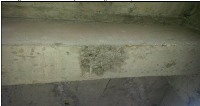
Fig. 7. Beam bottom found with traces of moss formation
