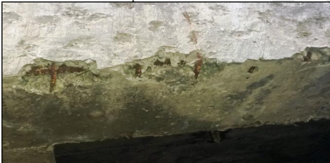
Fig. 6. Beam affected by broken edges and exposed reinforcement
