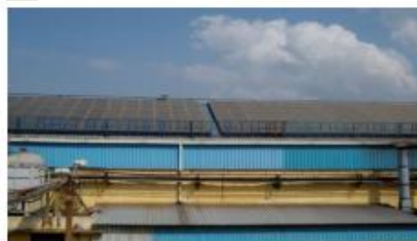
Figure6. Solar hot air for paint shop at manufacturing unit , Chennai, South India
