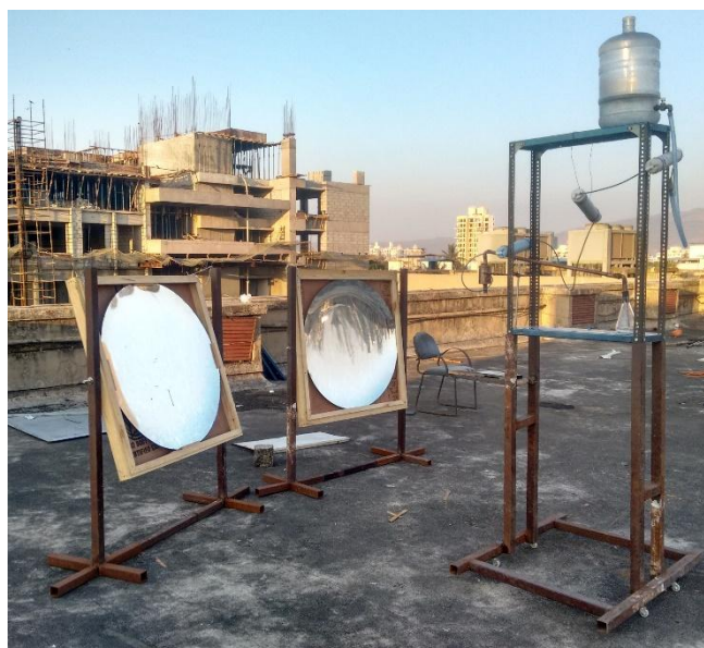
Fig. 5 Final Setup of solar Desalinator
