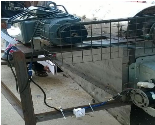
Fig. 10 Electrical connections (wiring and regulator)
