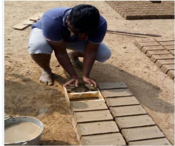
Fig 1 Moulding of bricks
