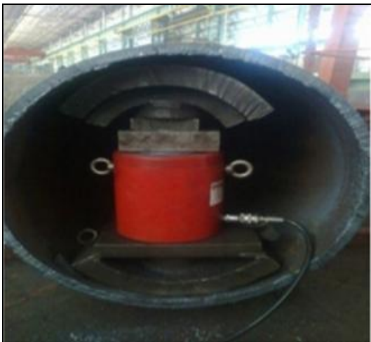
Fig.7. Ovality removal with the help of hydraulic jack
