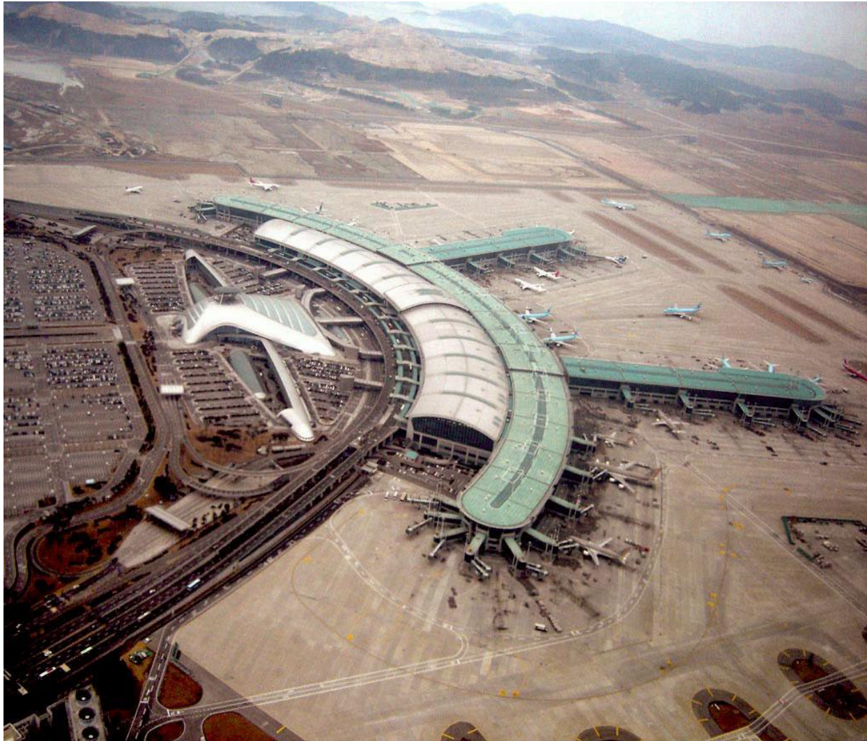
Fig. 1 Aerial view of Incheon International Airport in Jung-gu, Incheon, South Korea
