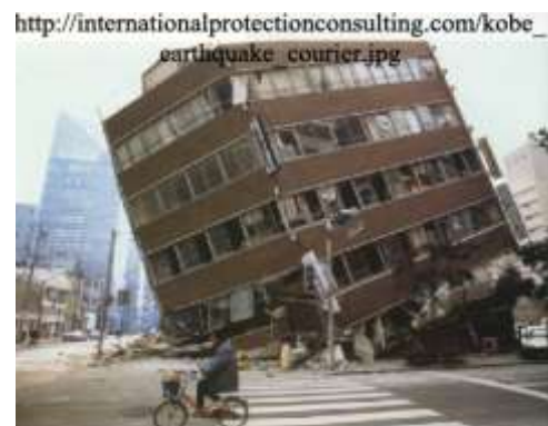
Fig.2 Collapse mechanism of a building structure having a soft storey
