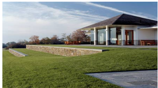
Fig.5 Zero House in Virginia, USA
