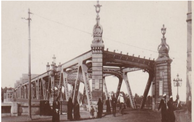
Fig. 4: Bridge May 15 th the present Alternative for Abul-Ela Bridge [5]
