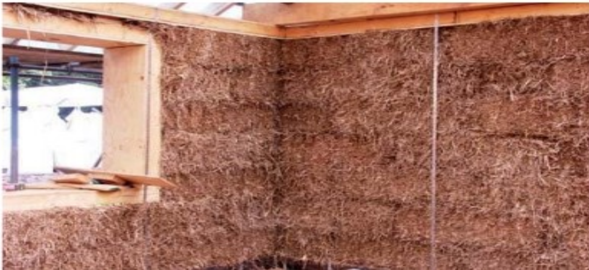
Fig 2 : The SSIM Mould wall under construction.
