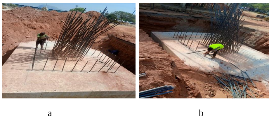
Figure 1. Schematic illustration of the post-installed rebar (PIR) system practical site work application: (a) Installed reinforcing bar embedded in hardened concrete using adhesive anchorage; (b) Sectional view showing the concrete, adhesive layer, and reinforcing steel bar.
