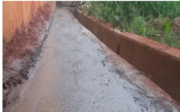
Figure 3: PKS pervious concrete walkway
