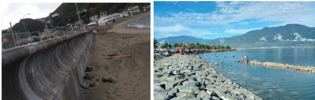
Fig. 9 Break water on Wellington and Palu Coastal[1]
